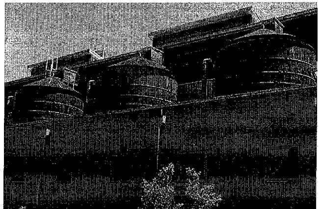
Cisterns at CBF headquarters. Photo: Chesapeake Bay Foundation.
