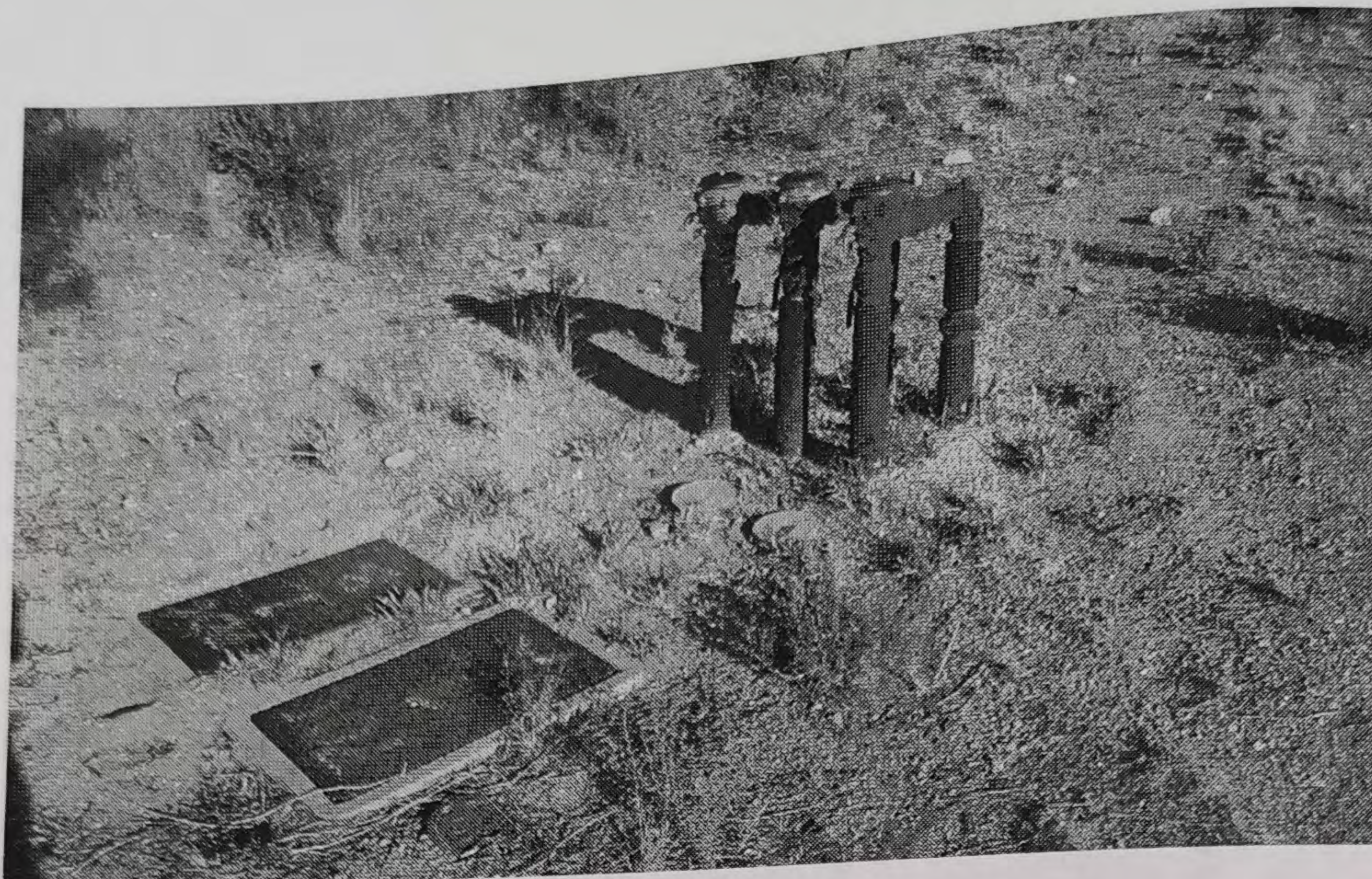
Figure 5-4: Atmospheric vacuum breaker
