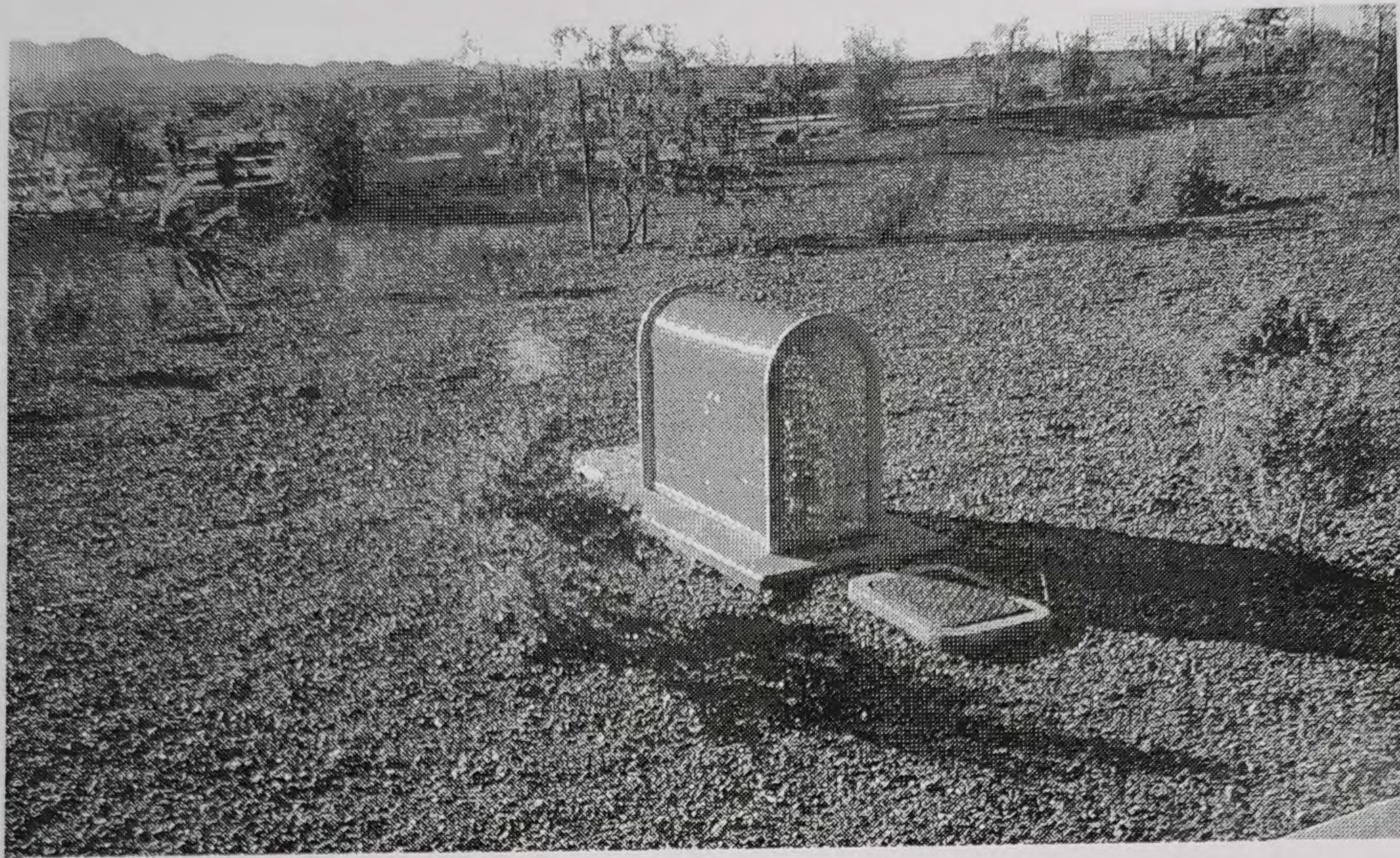
Figure 5-6: Backflow enclosure
