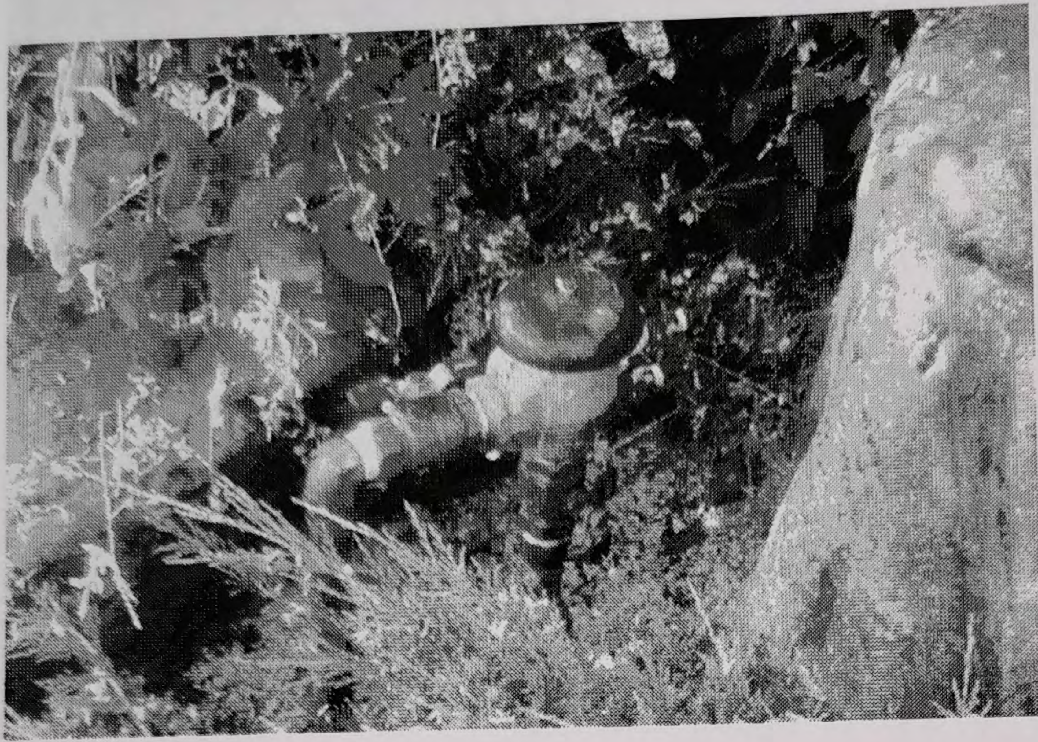
Figure 5-2: Pressure vacuum breaker
