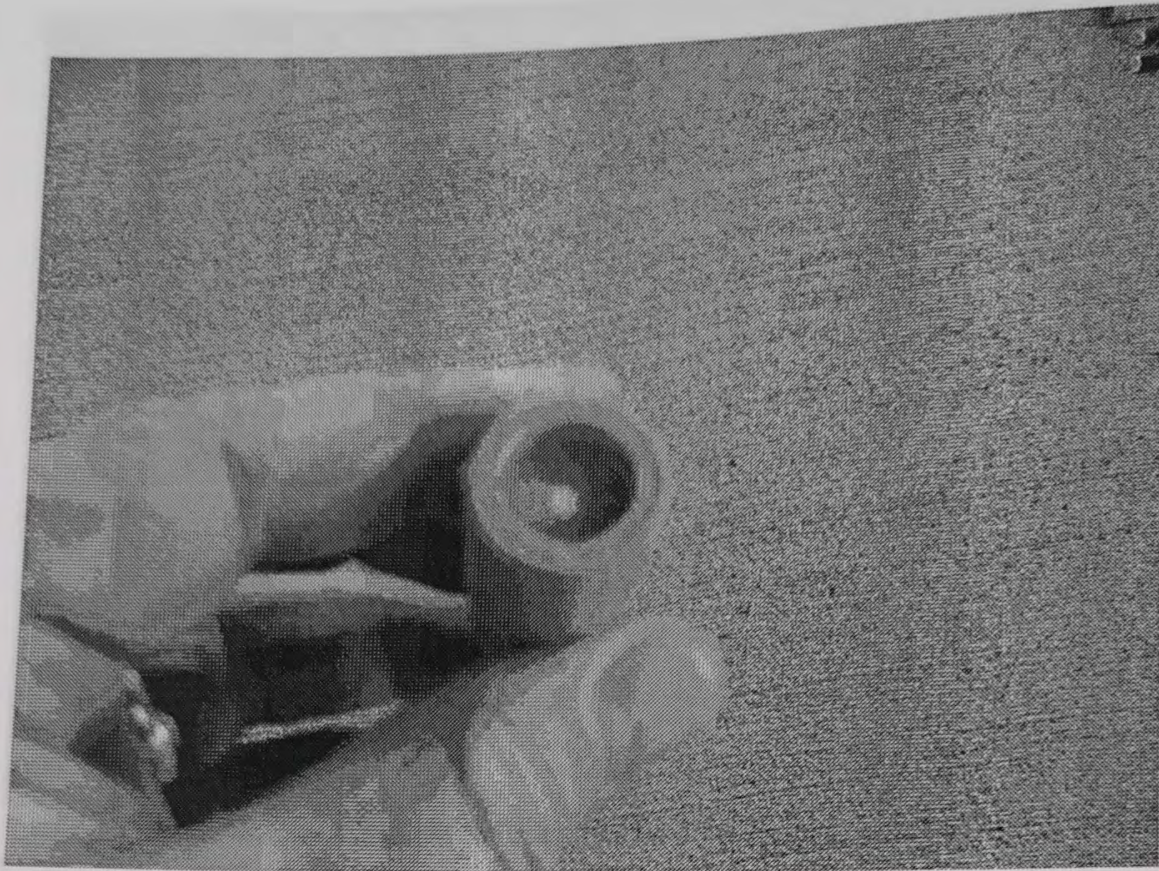
Figure 7-10: Splicing with waterproof filled wire nuts
