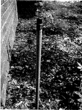
Figure 15. Shrub adapter with nozzle on PVC pipe nipple
