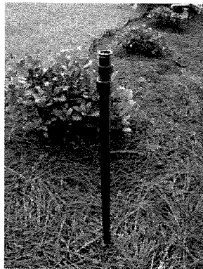
Figure 16. Shrub adapter with nozzle on PVC pipe with male adapter fittings
